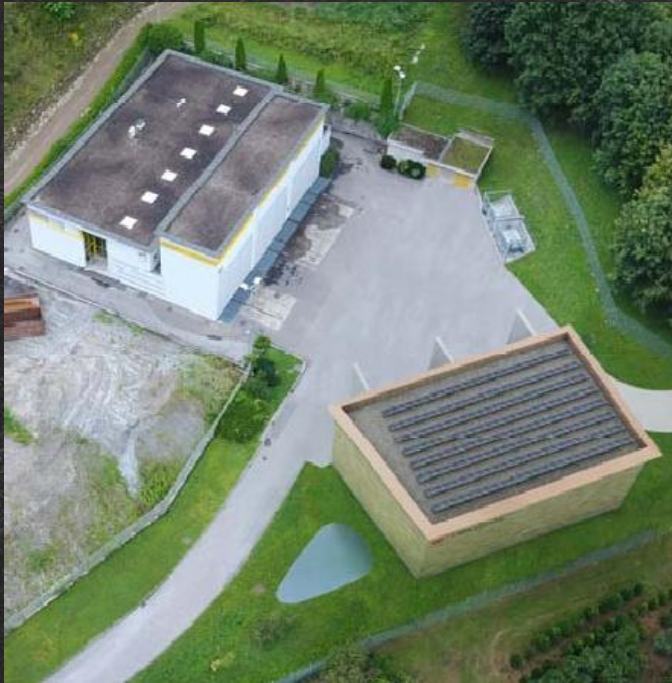
Version 1: Clay bricks with 3% cement (to stabilise the small format)
